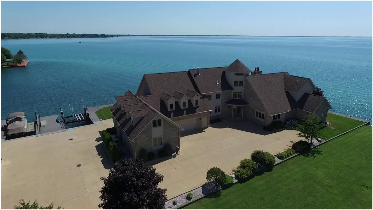
Other side of the same home looking toward the north-east at the same time as above.
